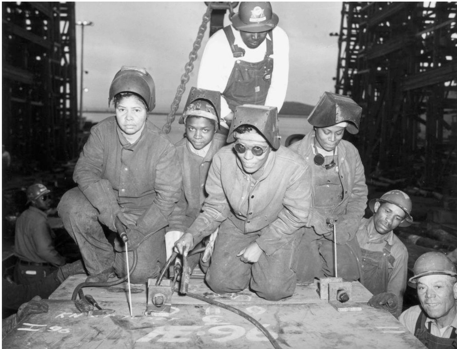
Richmond, California / Welders kneel in coveralls and hold tools as they prepare to work on SS ‘George Washington Carver,’ 1943 Photo by E. F. Joseph/Getty Images
