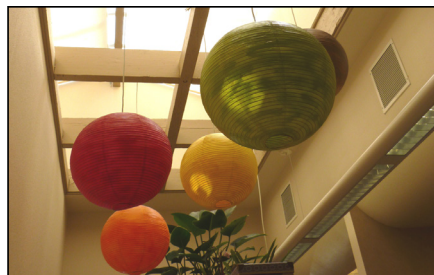
Natural skylight saves energy for lighting the office of Laura Lawson DDS
